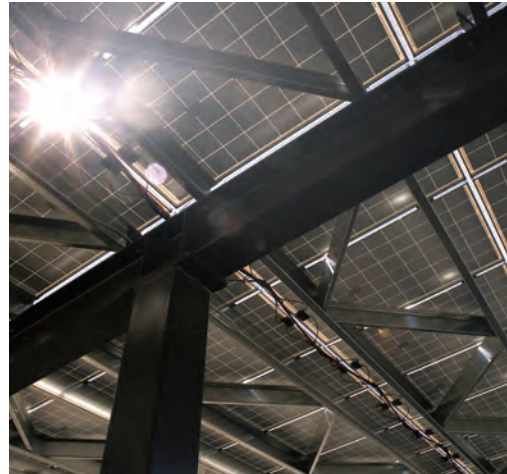
300 kW PV array canopies cover 50% of the parking lot
